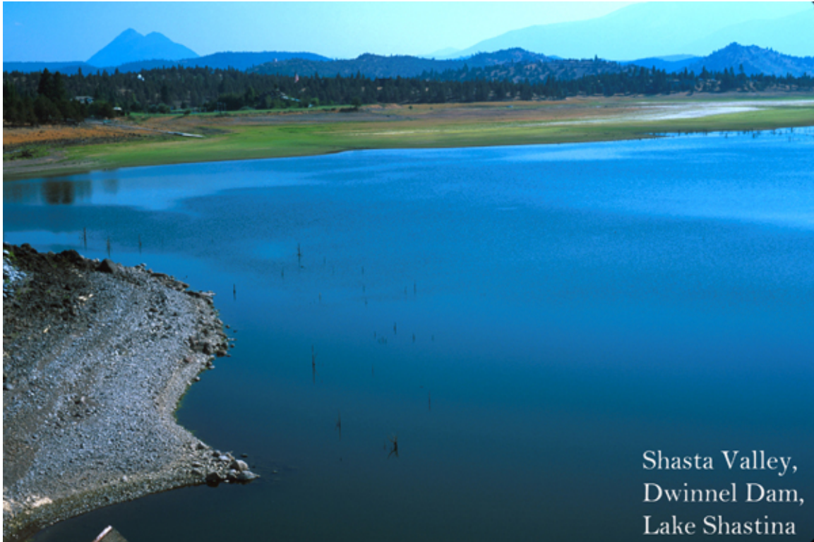
Figure 5. This photo shows Dwinnell Reservoir, also known as Lake Shastina, which has significant blooms of nitrogen fixing algae. Copyrighted photo used with permission of Michael Hentz.
